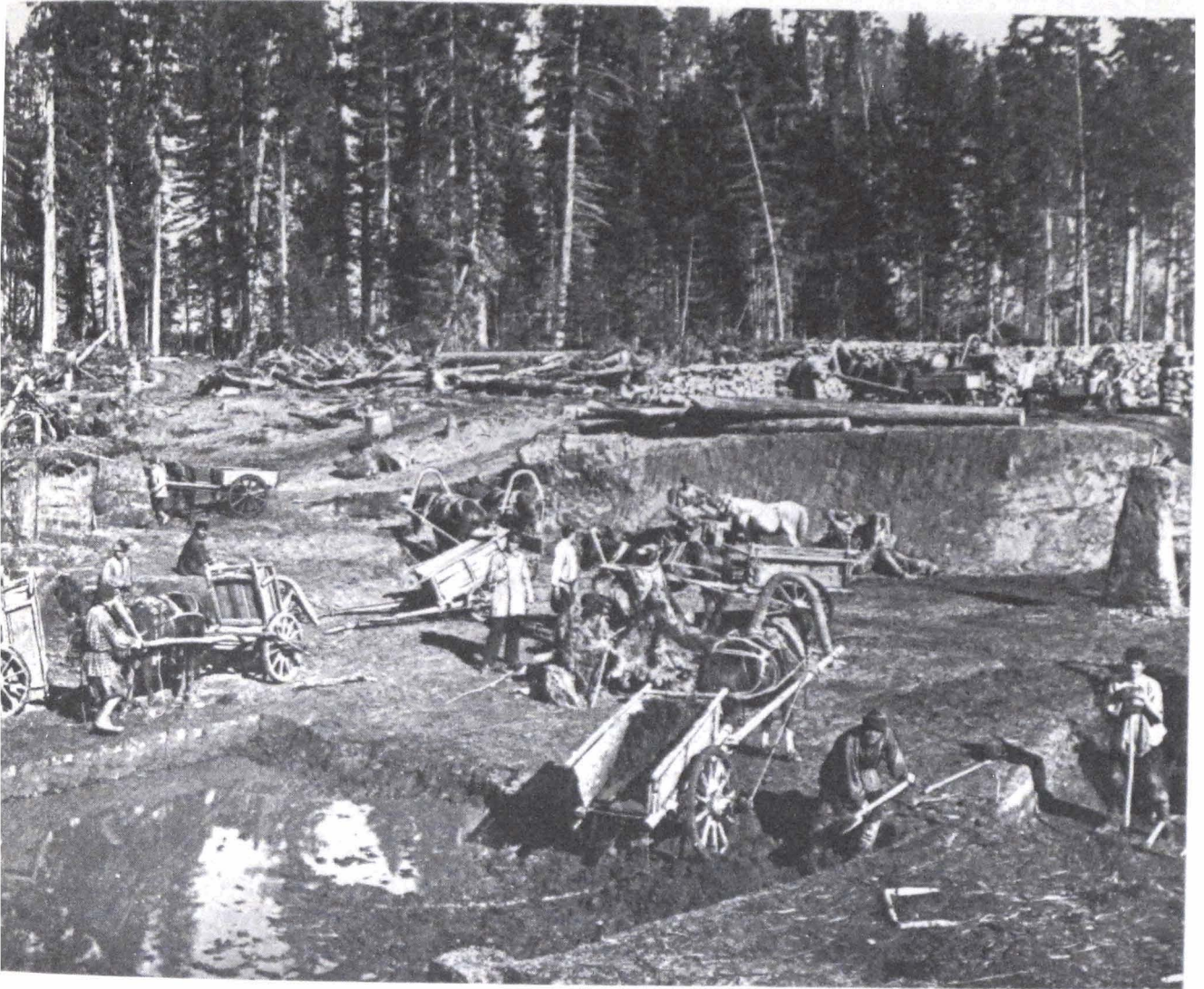
Unmechanized earthworks, Western Siberian line. From Velikii put': Vidy Sibiri i eia zheleznnykh dorog (Krasnoiarsk, 1899).
